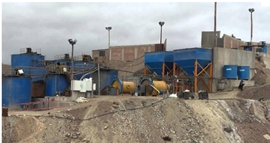
Chala One plant - North-west view
